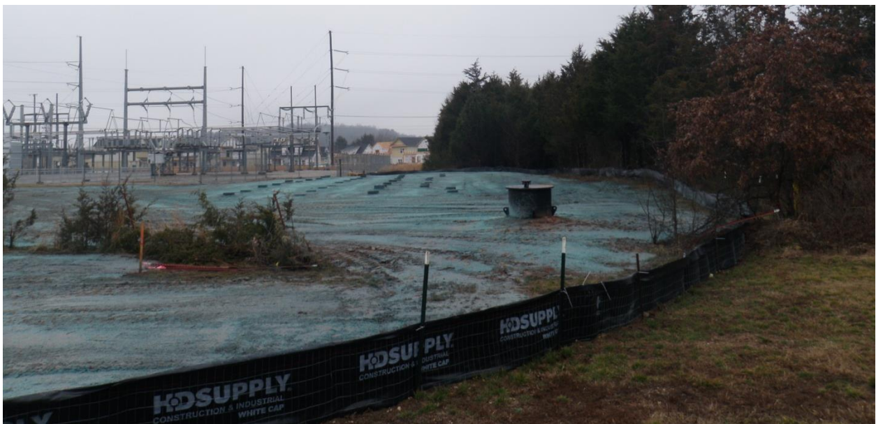
During: February 28, 2019, view from NW corner looking south toward injection wells and recovery well at the substantial completion site visit of Phase I.
